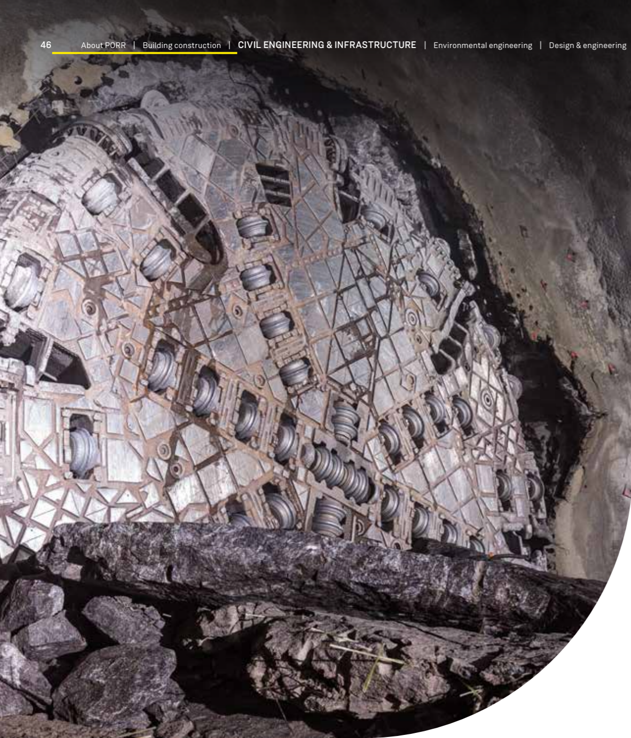
Drill head of a tunnel boring machine
