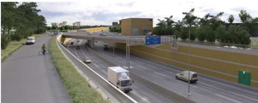
Photo: view over the completed cutting's structure and the flyover of Kiefholzstrasse / © ARGE SRB
